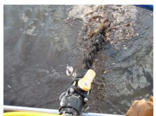
Muck is pumped from cylinder to firm bottom
